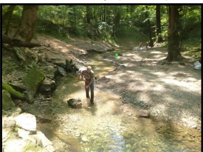
list for several years. Above ground, at Echo River Spring, was a stream bed where unwanted gravel (from previous Green River flooding) had been diverting and slowing the flow of water coming out of the cave, which affected the in-cave water level. The Resto Crew's job was to dredge gravel and reshape the path of the stream so that natural hydraulics would be restored.
